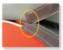
Finishing of stitching, that "covers" perimetrically the Velcro patches area to prevent case and patches from getting torn.
